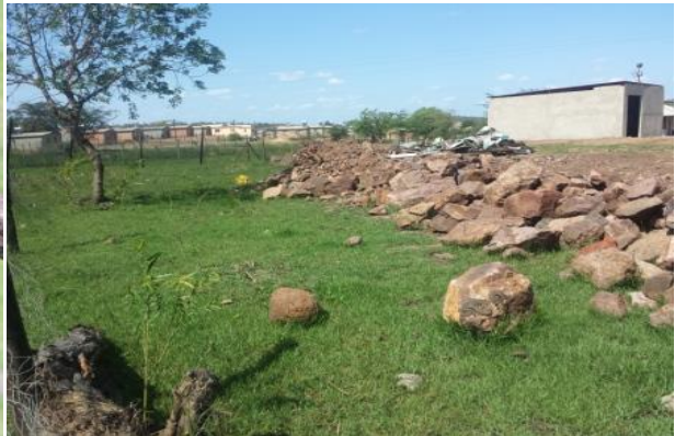
Photo 2: View showing the edge of Wetland Unit C1-W02 which has been infilled with earth and rock to construct a housing platform.
