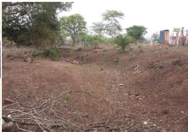
Photo 4: View looking up-stream of the culvert showing the dry river bed.
