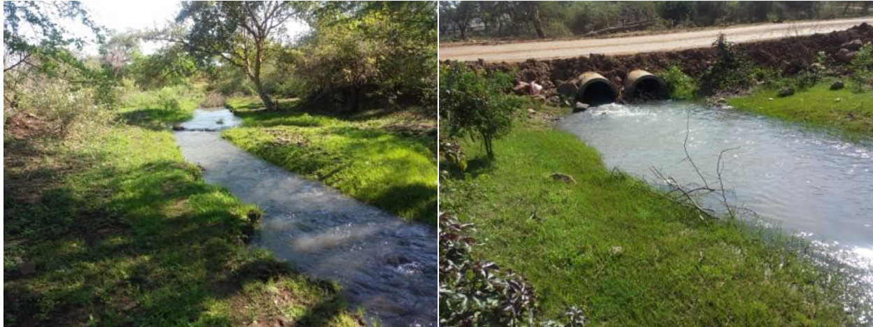
Photo 5: View looking downstream of the wetland showing an active, flowing channel (culvert 3) Photo 6: Outlet of culvert 3 to be replaced.
